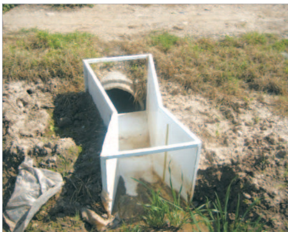
Fig. 1 Installed cut-flume in selected fields of Sorkheh site.
