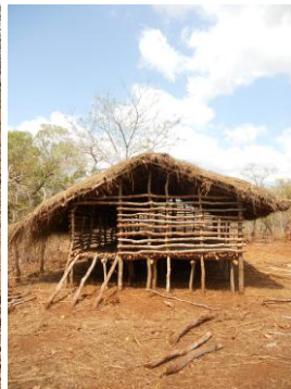
Figure 5: lateral view of shelter (unfinished)
