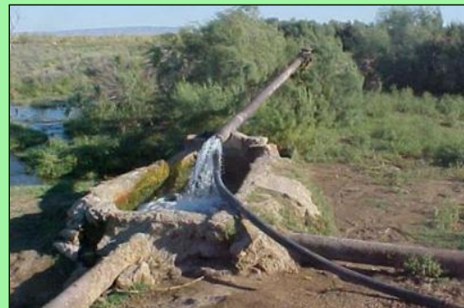
Figure 1. A general view of an artesian well and a water intake for irrigation (Photo by: A. Rabbimov)
