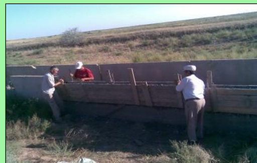
Figure 1. Reconstruction of irrigation canal by local community for autumn and early-spring irrigation of alfalfa from the Talas River (Photo by: Gulnara Bekturova)
