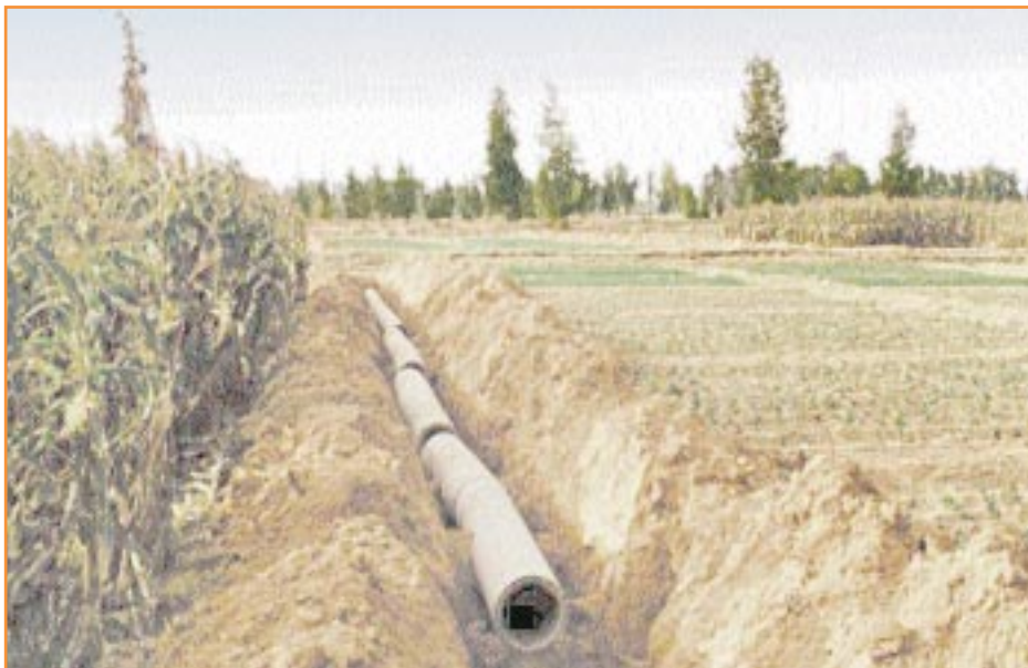
Mole drainage systems establishment in El-Serw on salt-affected old land in the lower Nile Delta.
