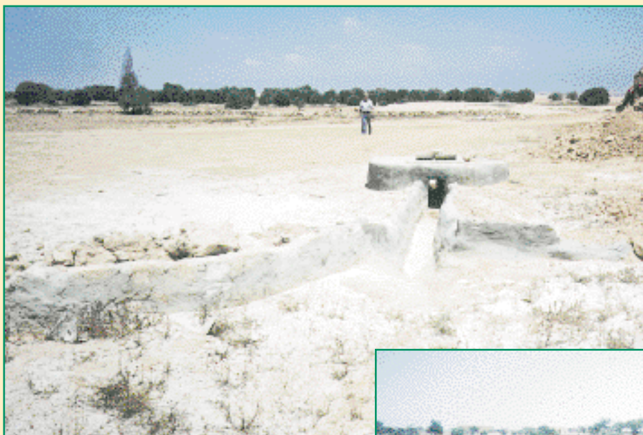
Above: Cisterns are an ancient technology being put to good use by the Matrouh Resource Management Project. A large tank of mortar and stone stores rainwater caught in natural and man-made channels.
