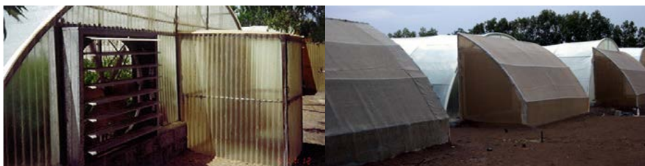
Figure 7 - As part of the IPPM package, using double doors and covering all ventilation with insect proof net are widely accepted and adopted in UAE
