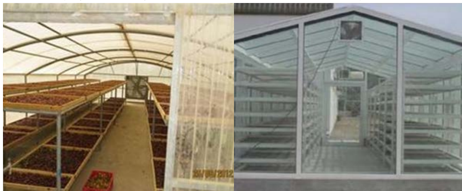
Figure 8 - Glass (left) and Polycarbonate (right) drying dates houses
