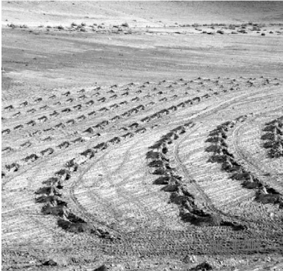
**Fig. 3** Constructing Vallerani micro basins of different sizes on the contours of different slopes (Badia, Jordan).
