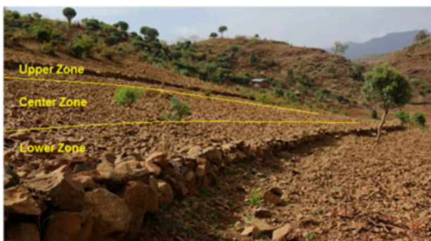
FIGURE 3 Investigated stone bunds in the Gumara-Maksegnit watershed showing upper, central, and lower zone of stone bunds. Trampling path just below the stone bund can be seen [Colour figure can be viewed at wileyonlinelibrary.com ]
