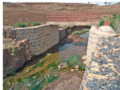
Figure 8.2 Main outlet gauging station of the Gumara-Maksegnit watershed (pressure transducer and turbidity meter are installed at the right side wall of the fixed cross section at \approx 20 cm level above the channel bed)
