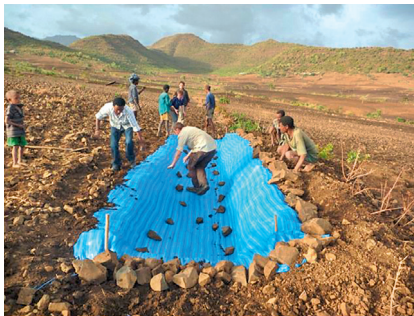
Figure 8.8 Design of the erosion ditch at the outlet of the treated hill slope
