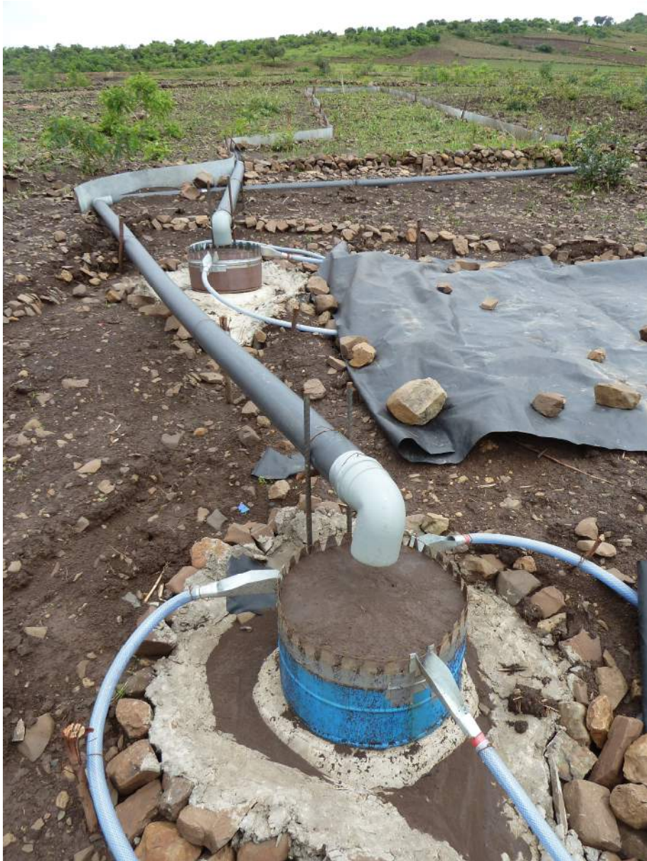
Figure 15: Treated plot, ready for operation
