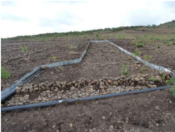
Figure 19: Stone bund before maintenance
