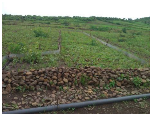
Figure 18: Stone bund after maintenance
