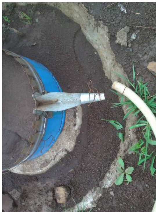
Figure 39: Removed connection tube between the sample divider and the pond of the UT plot
