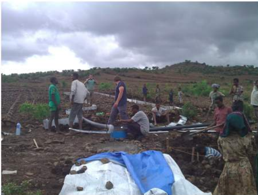
Figure 9: Construction works for the plots
