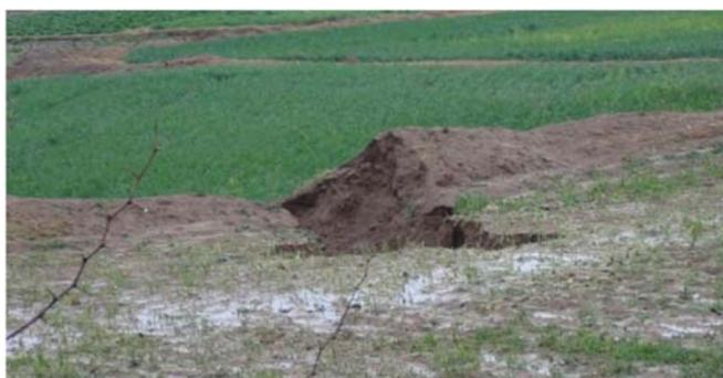
Figure A2 Breached terrace bund/embankment
