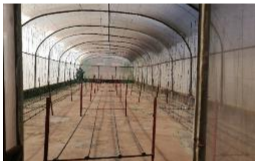
Figure 5. Screenhouse emptied and rehabilitated.
