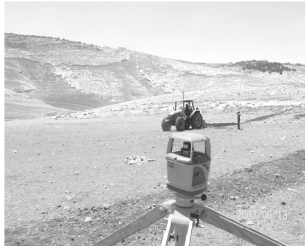
Fig. 2 The laser beam transmitter mounted on a tripod on uphill side.
