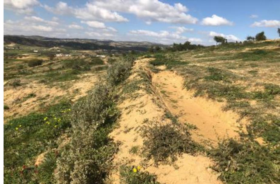
With a total distance of 700 m and a water retention capacity of  $0.4\text{m}^2/\text{m}$ , a total estimated water harvesting is expected to be  $280\text{ m}^3/\text{year}$
