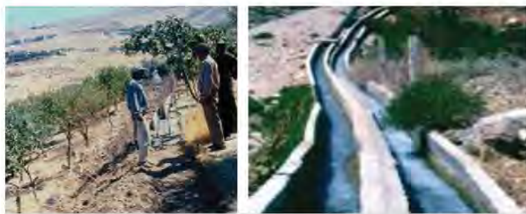
Large amounts of water are lost from unimproved irrigation canals (left). Concrete-lined canals (right) and plastic pipes avoid these losses, delivering more water to the farmers.
