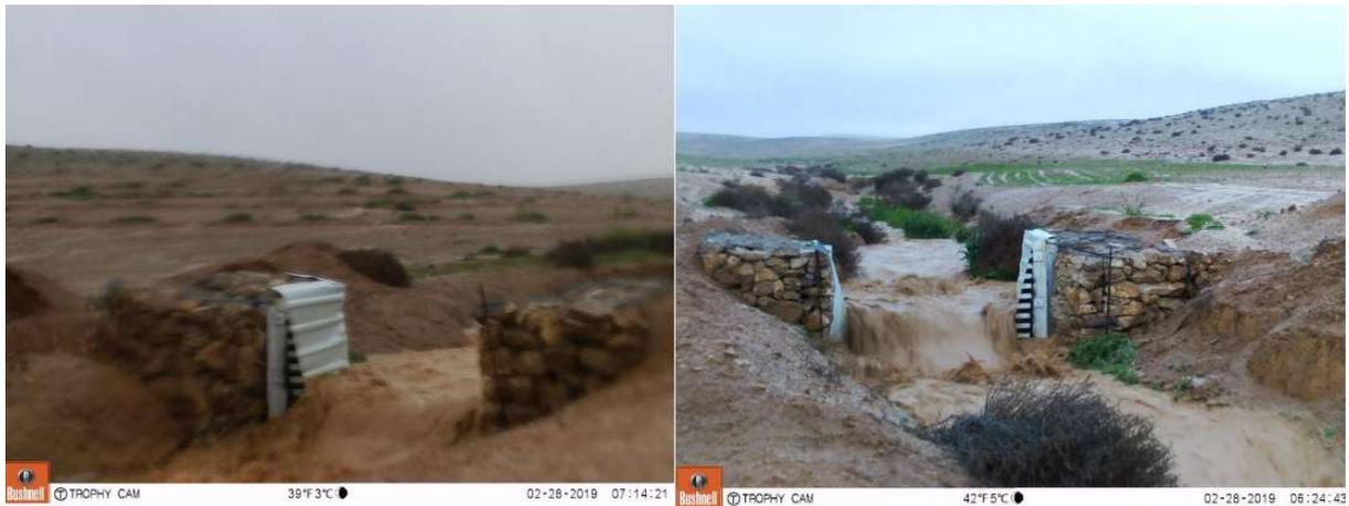
Figure 9: Run-off event of 28<sup>th</sup> February 2019 for untreated gully (right) and rehabilitated gully (left) (Goos, 2019)
