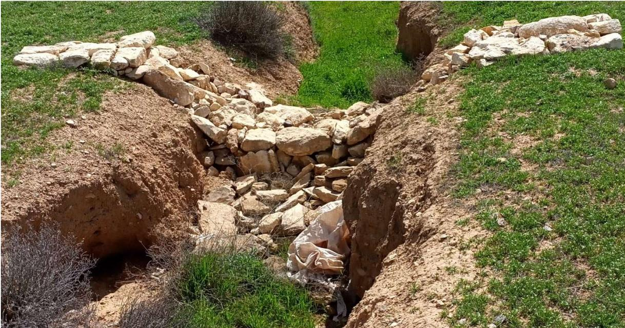
Figure 8: Picture of a stone gully plug with flourishing vegetation and trapped sediments (Verbist, 2020).
