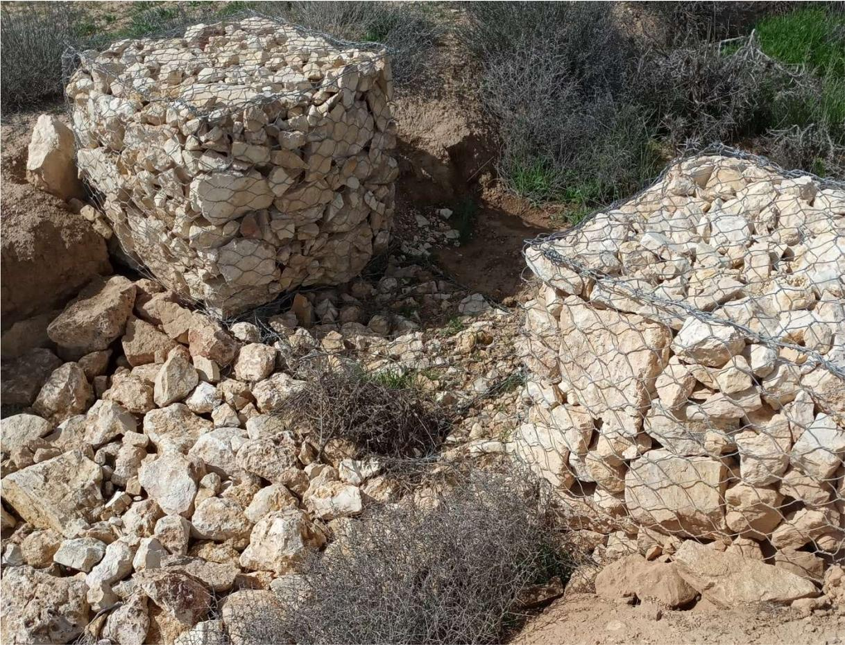
Figure 7: : Picture of a gabion gully plug (Verbist, 2020)
