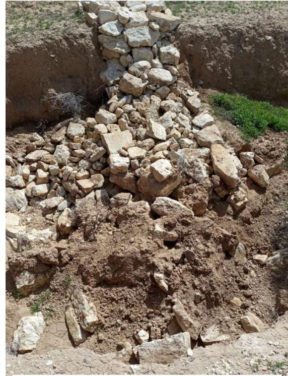
Figure 19: Picture of a failed gully plug (Verbist, 2020)
