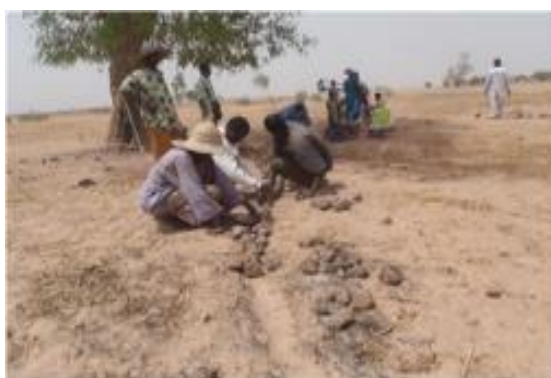
Construction of stone barriers (photo: JICA)
