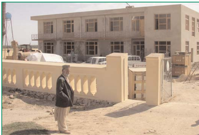
Rehabilitated research station in Baghlan.
