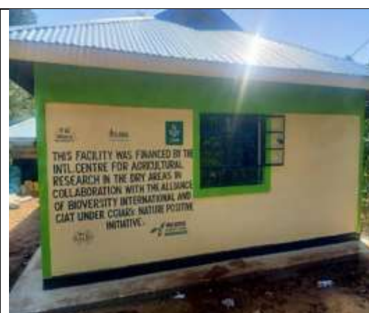
Figure 7. Vihiga seed processing facility
