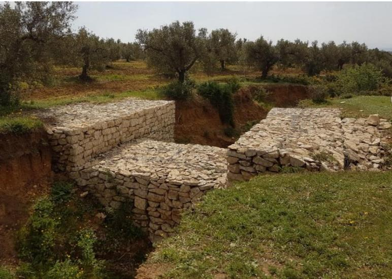
It is a structure built of uncemented stones but well anchored on the banks in order to increase its cohesion and rigidity.
