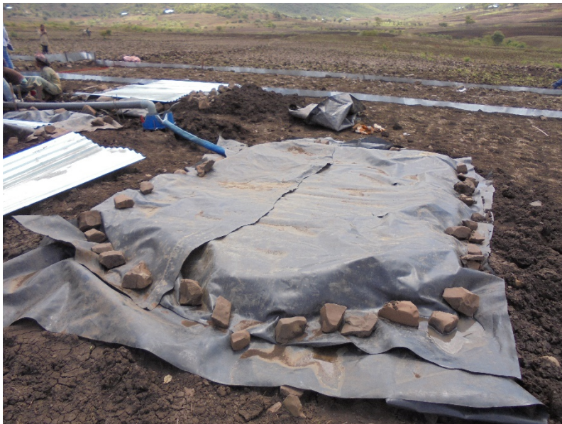
Figure 4-9: Collection pond covered with corrugated iron sheet, plastic foil and stones (photo: E. Obereder)
