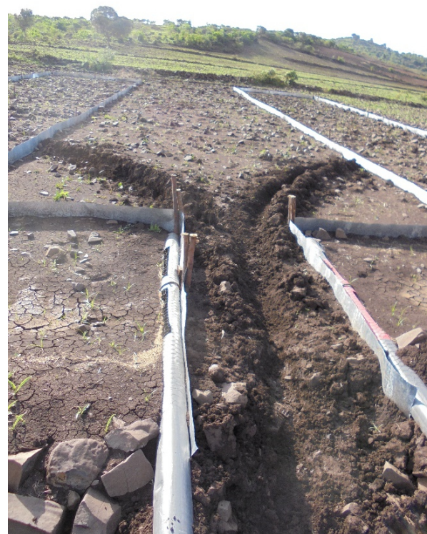
Figure A.1-1.2: Spillways to divert the surface runoff (photo: E.Obereder)
