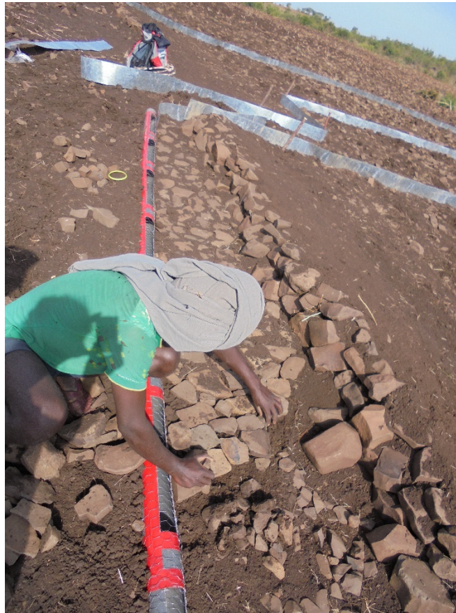
Figure 4-6: Installation of stone terraces (photo: S. Wakolbinger)
