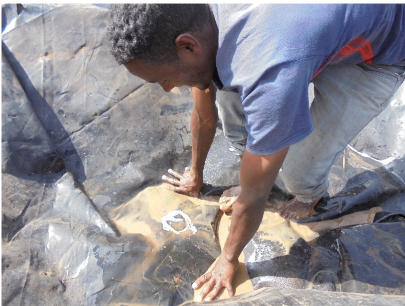
Figure A.1-1.1: Hole in plastic foil at TP 1 – SF (photo: E.Obereder)
