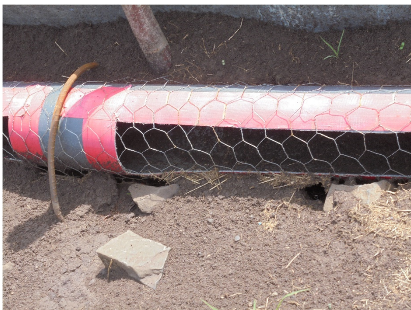
Figure A.1-2.1: Holes underneath the collection pipe (photo: E.Obereder)
