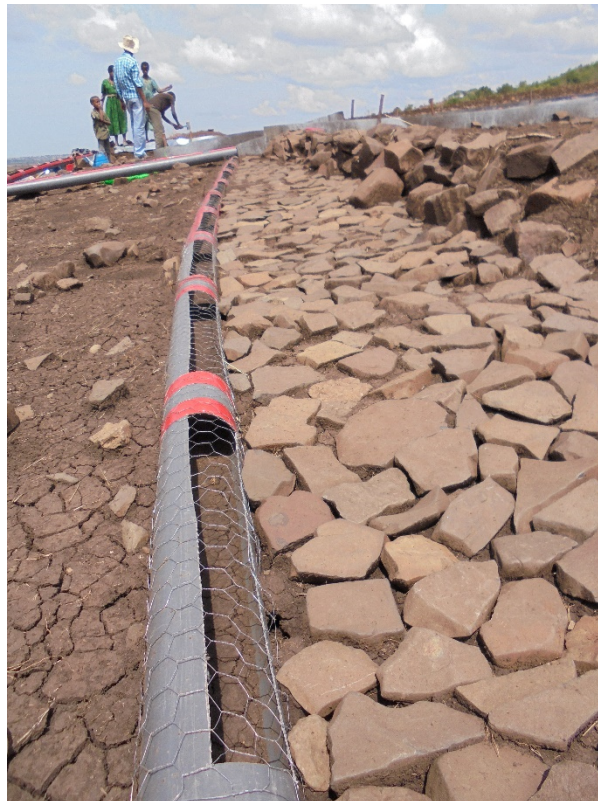
Figure 4-5: Collection pipe with mesh wire cover (photo: S. Wakolbinger)
