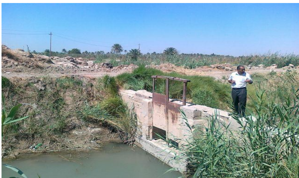
Figure 4: View of typical regulators to control flows in the irrigation canals.
