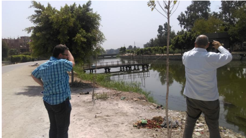
Figure 9: Drinking water intake station on Abul Akhdar Canal
