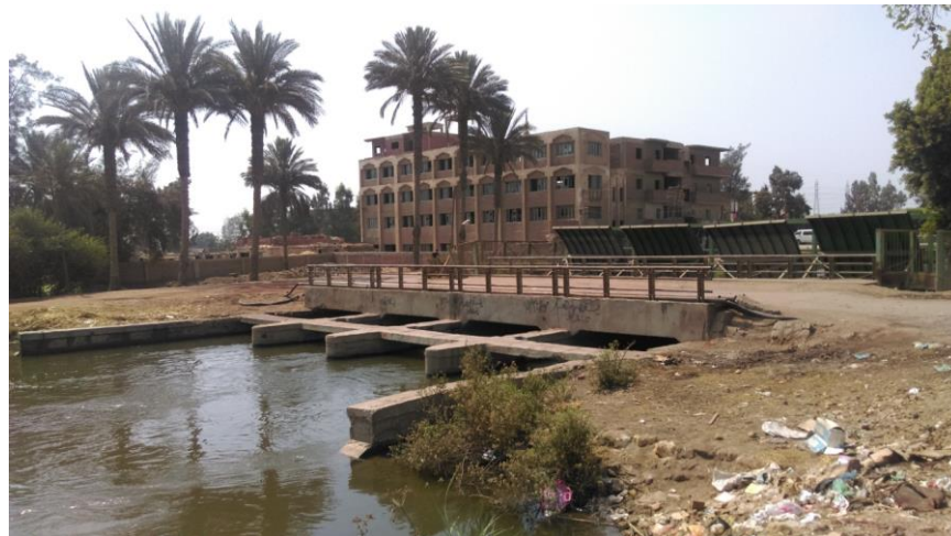
Figure 7: Regulator on Abul Akhdar Canal
