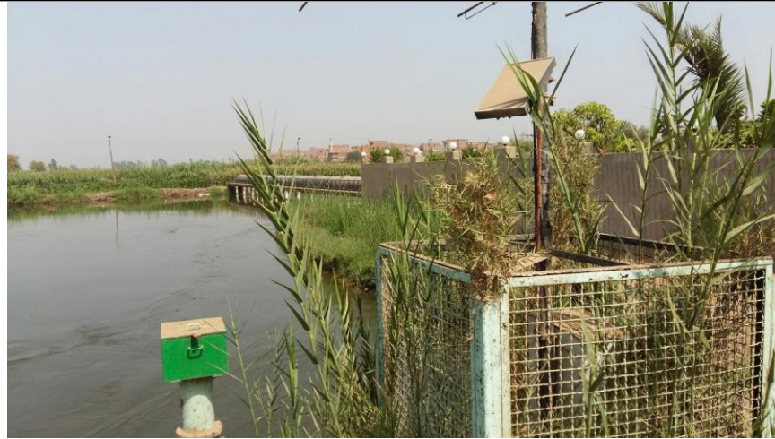
Figure 6: Telemetry station at the intake of Abul Akhdar Canal
